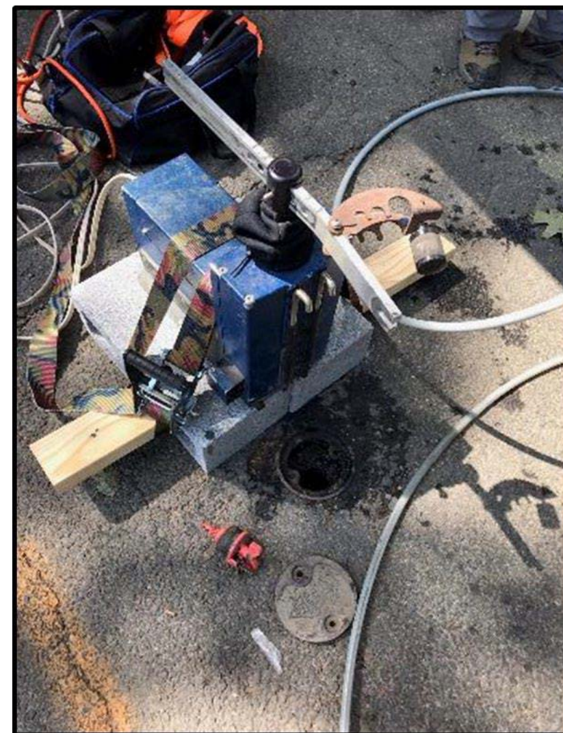
Groundwater sampling well
